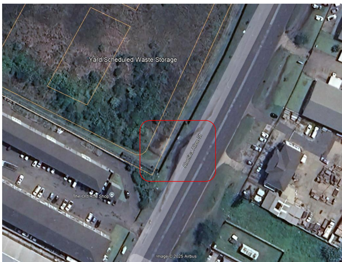
Figure 7-1: Potential stormwater pooling on Alumina Allee Street
